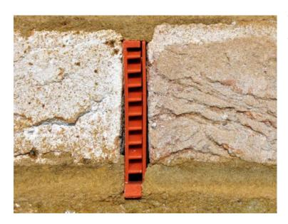
Weep vent to allow the transit of water, to expel onto outer wall, to maintain a dry cavity (picture for illustration purposes only).
